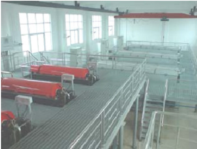
The installation in the Chandong WWTP;
