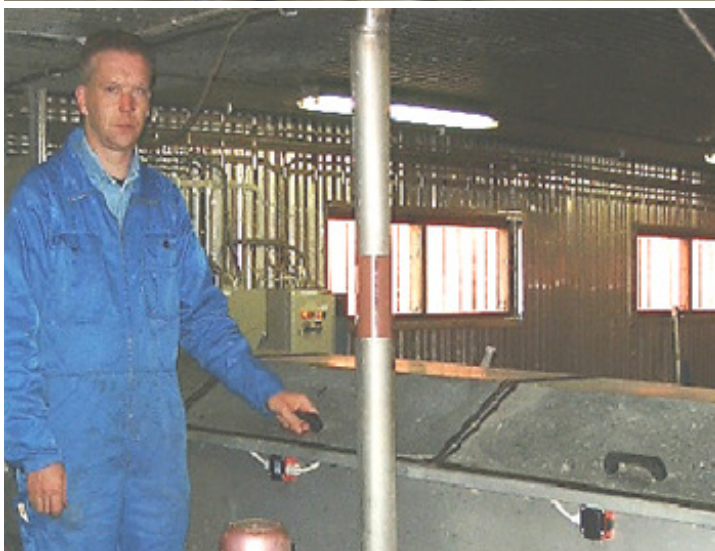
A very pleased chief operator at Rättviks waste water treatment plant, standing next to their Siljan RotoMaster SF17. The installation was performed in year 1998, to thicken sludge entering a digester. A Siljan PolySave was also installed during year 2000. The combination Siljan RotoMaster and PolySave gave significant cost savings concerning heating requirement, operators attention and polymer consumption. A significant increase in gas production was also achieved.
